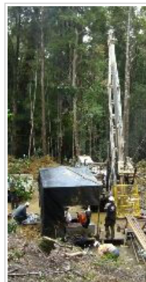
Drilling at Venture Minerals' Mt Lindsay project
