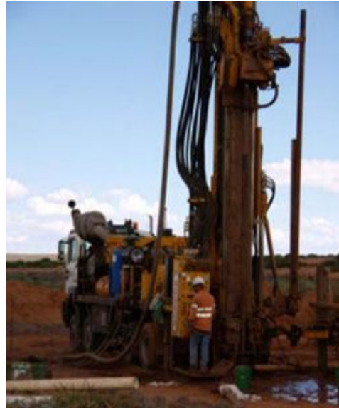
Venture Minerals drilling operations
