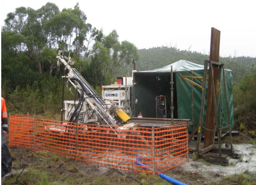
Drilling hole LV001 at Stanley River
