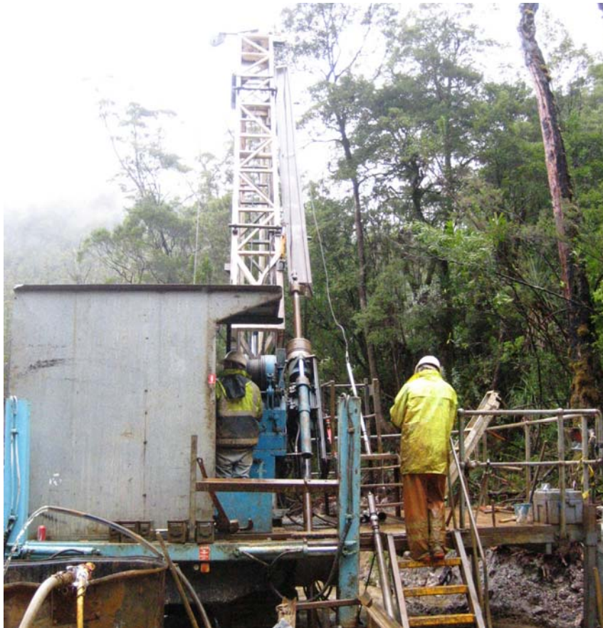
Drilling at Stanley River
